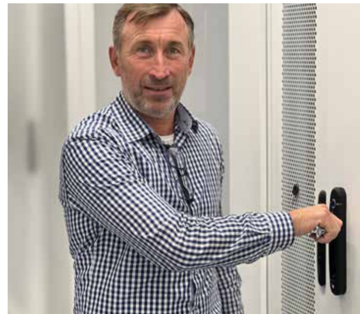
The individual doors of the server cabinets are secured using the "Agent E Wireless" system supplied by EMKA.
