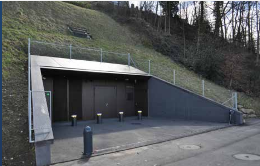
The old civil defence bunker in the Wartegg hill near Lucerne was converted into one of the most modern data centres in Switzerland.
