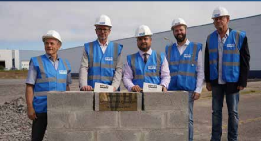
The groundbreaking ceremony for the new building project took place on 14 September 2023.
