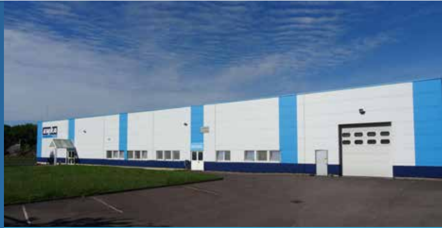
EMKA France Fort doubles the production area at its Henriville site with a new production hall.
